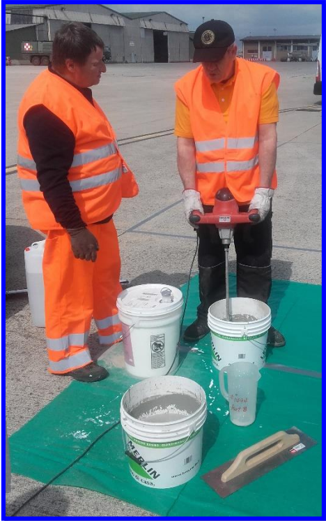
Mixing of the polymer, water and concrete
