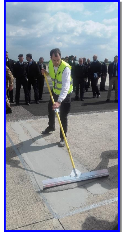
Final thickness of the application: 0,7/0,8 mm
