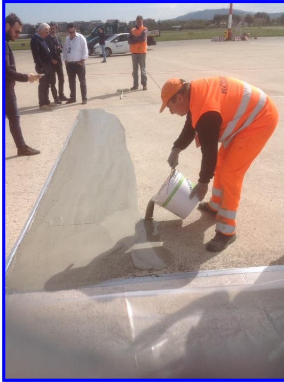
Application of the mix in two consecutive layers
